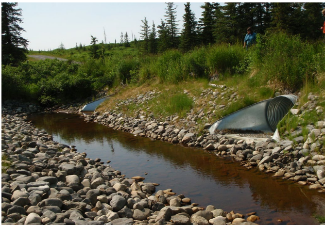
New fish culverts (2013), Ninilchik Native Association
