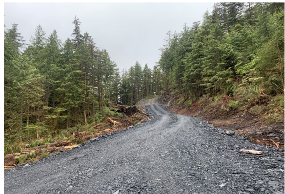
Road reconstruction Keete Inlet
