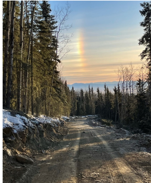
New road construction, AKA Maisch Logging Road, connecting Parks Hwy to Upper Grouse Rd. (Kevin Meany)
